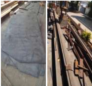
Road construction equipment (MS plates and channels)
