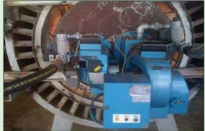
(Fig. 4b: View of the Gas Burners (2 Nos. to match the heat energy input) fitted on the DF heater)
