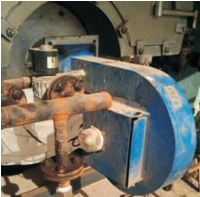
Low efficiency single stage burner
