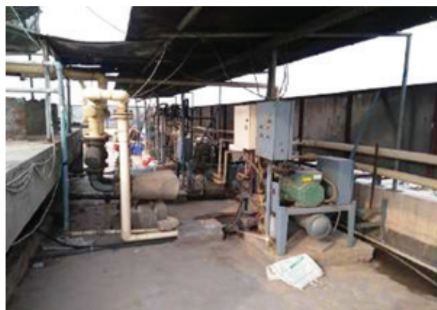
Refrigeration compressors: screw compressor
