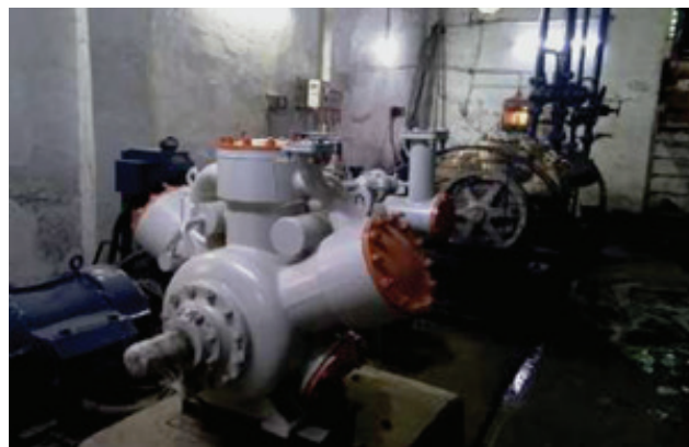
Refrigeration compressors: reciprocating ammonia compressor
