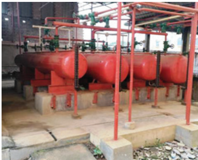
Ammonia tanks in a cold storage facility
