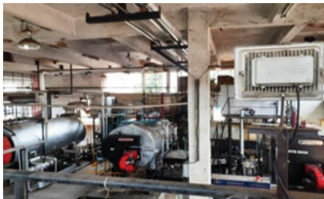
Installed boilers in dairy plant
