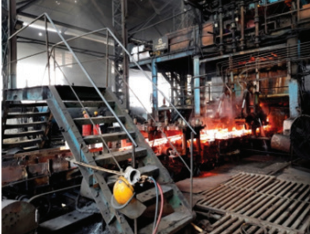
Steel melting industry: continuous casting machine (CCM)
