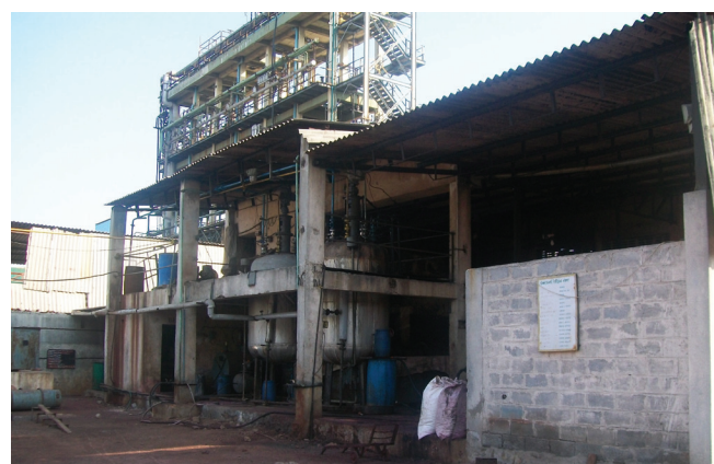
View of chemical unit
