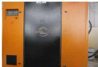
Replacement of reciprocating air compressor with inverter type screw air compressor
