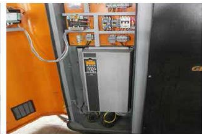
Replacement of reciprocating air compressor with inverter type screw air compressor
