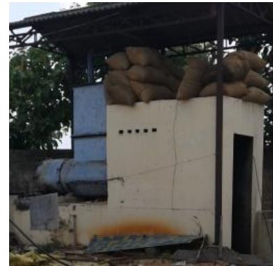
Rice husk fired boiler
