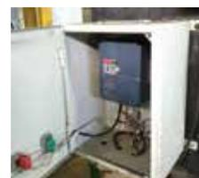
VFDs installed in motors
