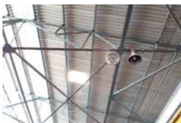
*Conventional lamp replaced with induction lamp*
