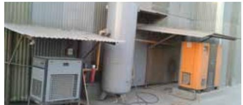
*Screw air compressor with a receiver and dryer*
