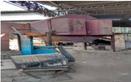
Waste heat recovery system
