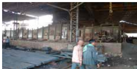
Pusher hearth reheating furnace
