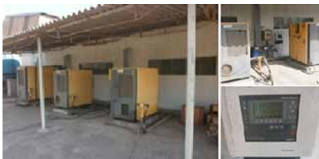
(L) Air compressor system; (R) with sequence controller
