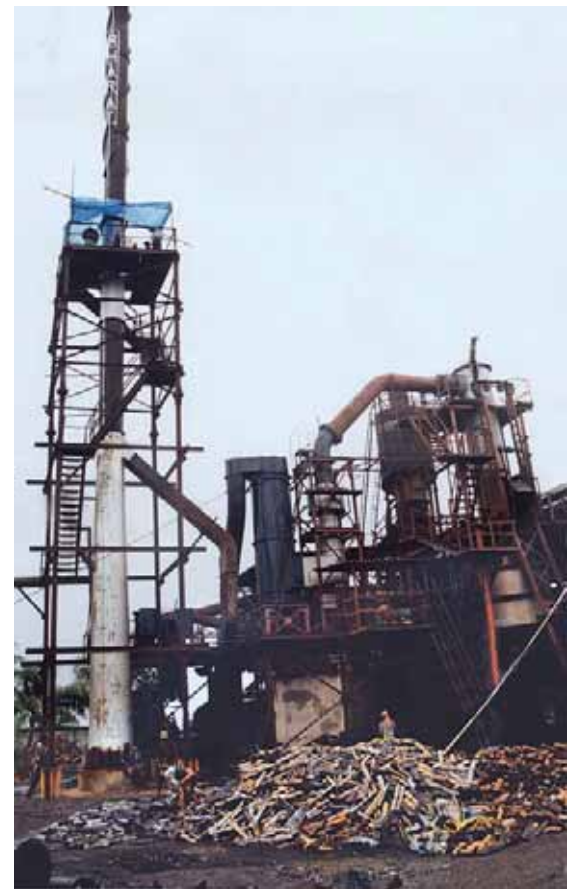
Demonstration plant at Howrah
